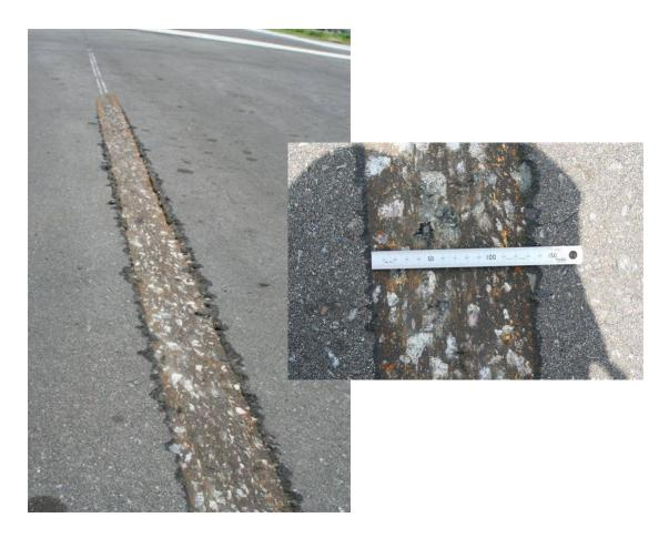
Figure 4: Nose landing gear scrape on runway approximately15 cm wide
